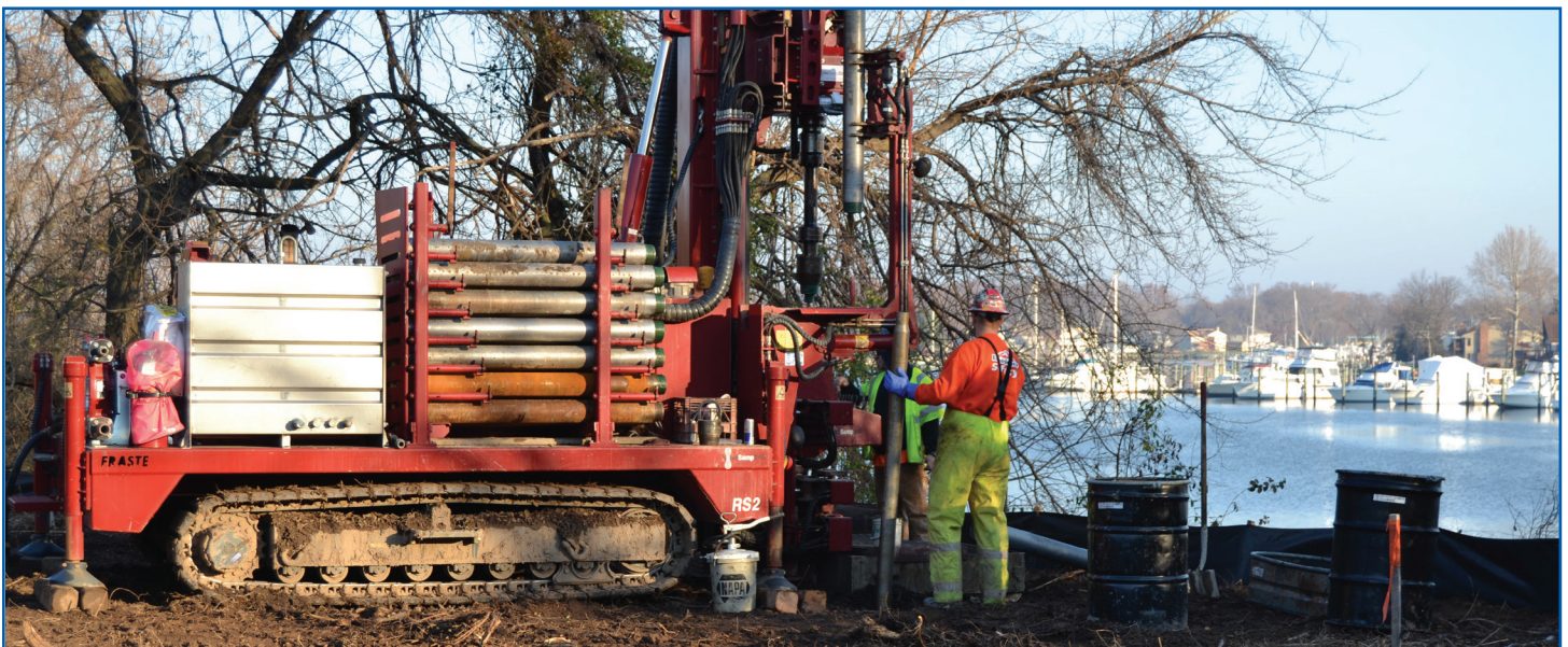
Drilling of initial extraction well borings began in December 2015.
