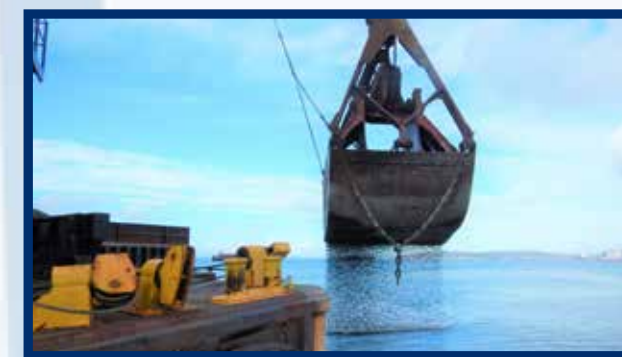
Fill placement complete: February 11, 2020
