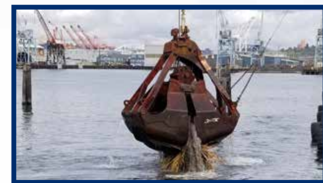
Main Dredging Complete: November 25, 2019
