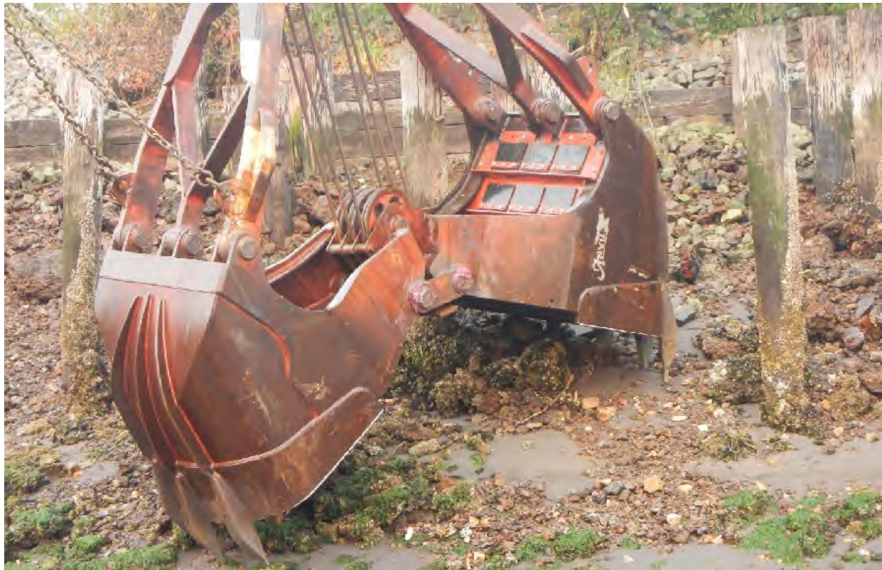
Photo 4 Removal of Shoreline Debris Using Dredge Bucket
