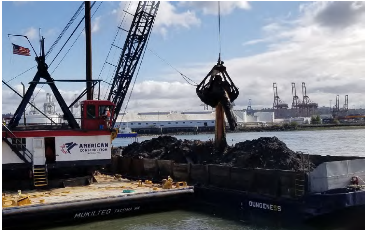
Photo 6 Standard Digging Dredge Bucket Used in Areas of Significant Debris or Dense Sediment
