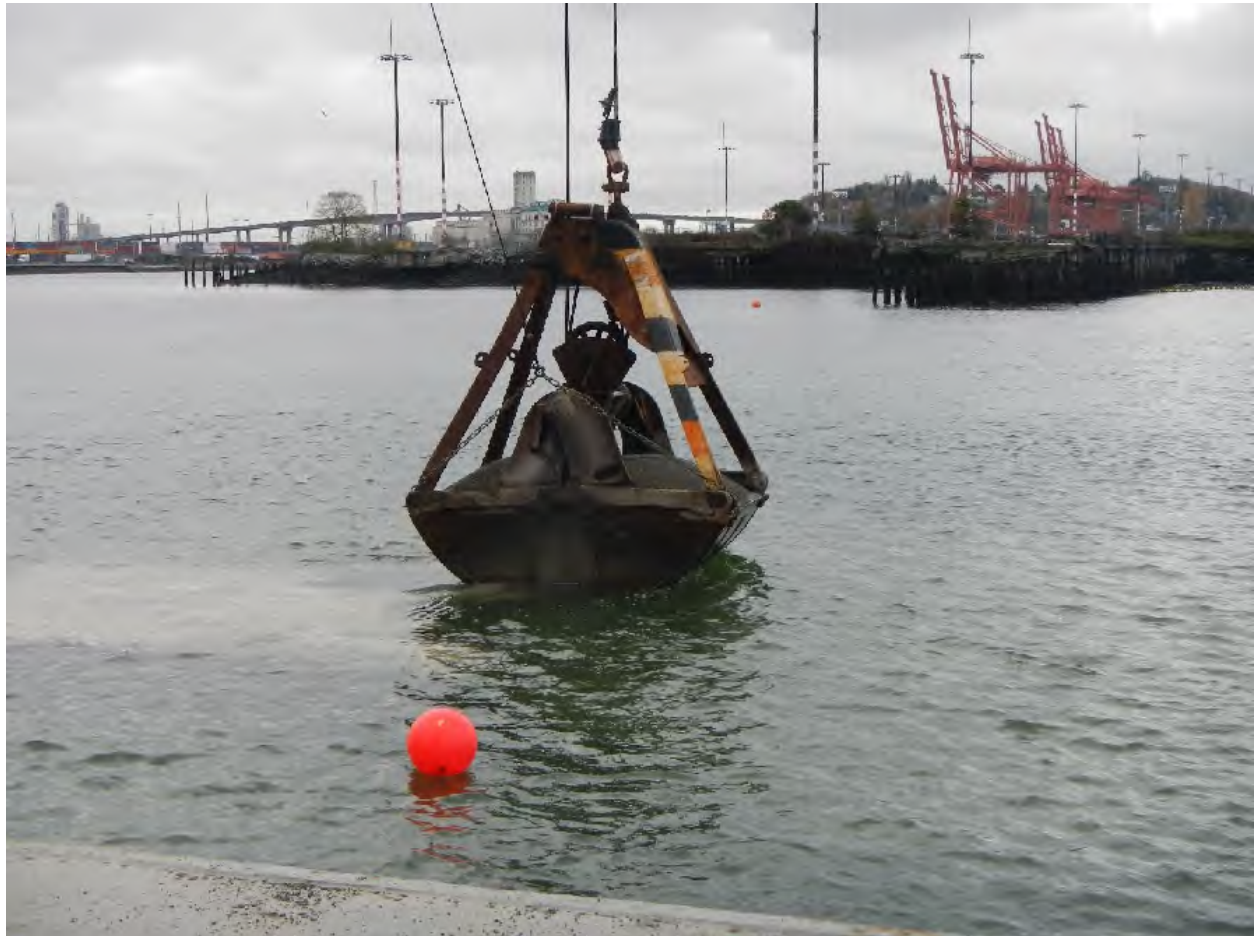
Photo 10 Placement of Residual Management Layer
