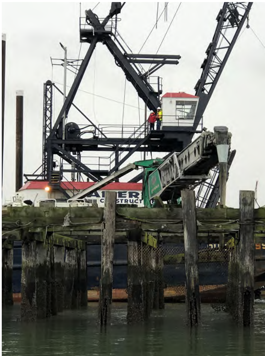
Photo 14 Placement of Enhanced Natural Recovery Layer by Telebelt
