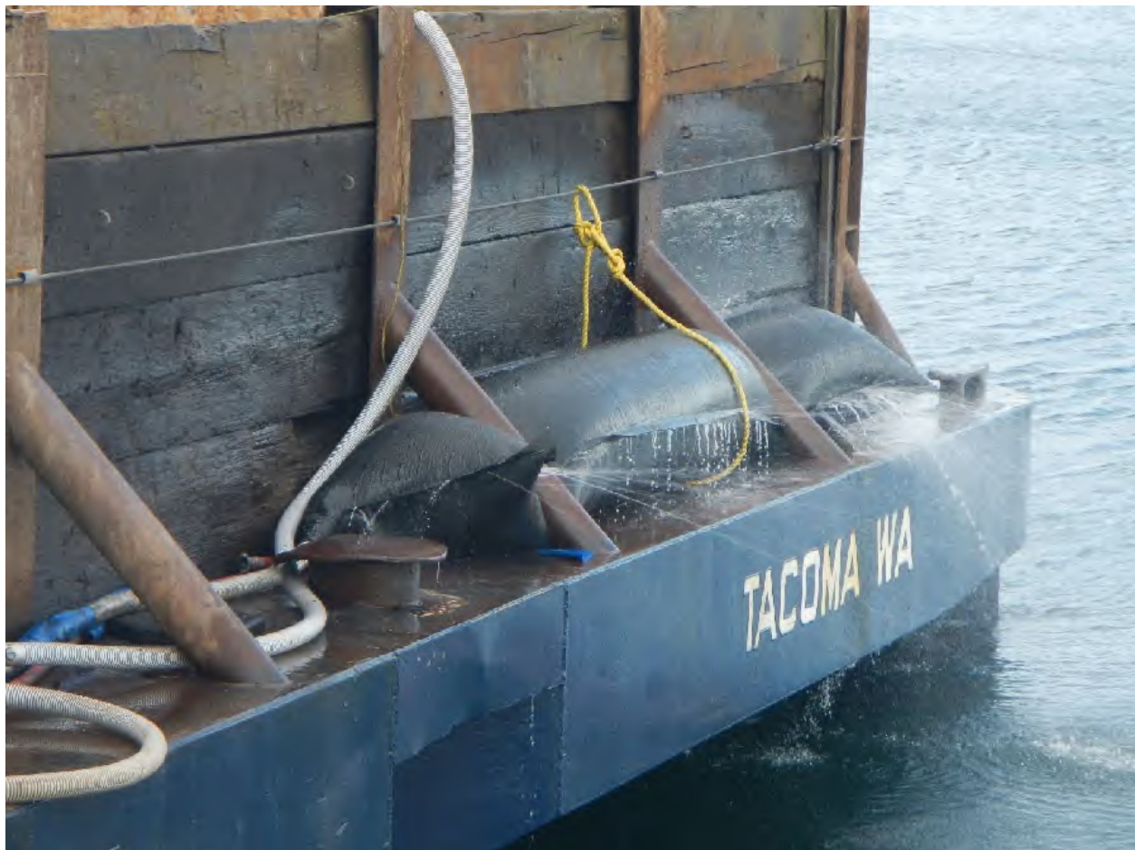
Photo 7 Geotextile Filter Bag Used Prior to Discharge of Dredge Return Water
