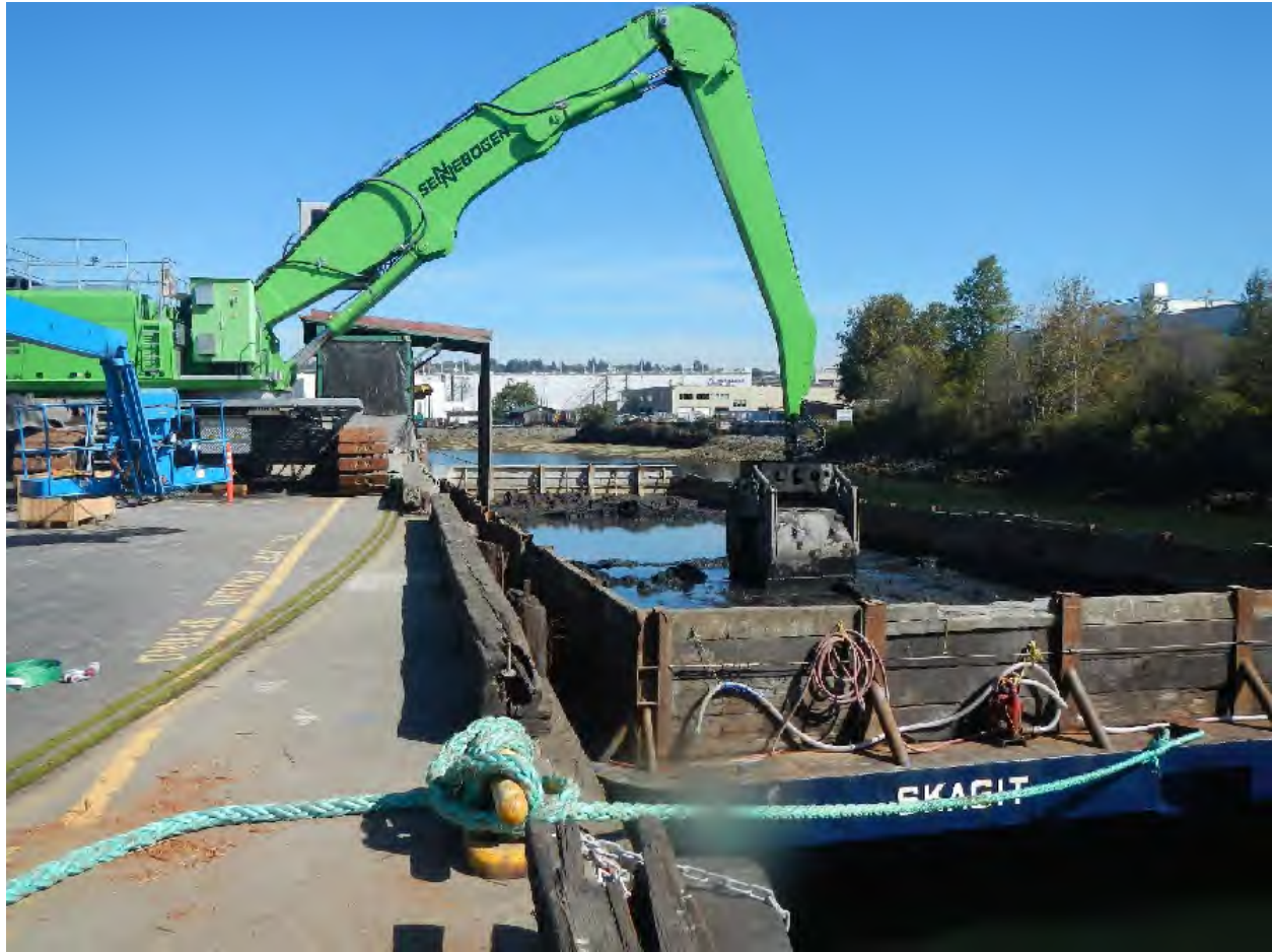
Photo 15 Uploading of Dredge Material from Barge at Reload Facility
