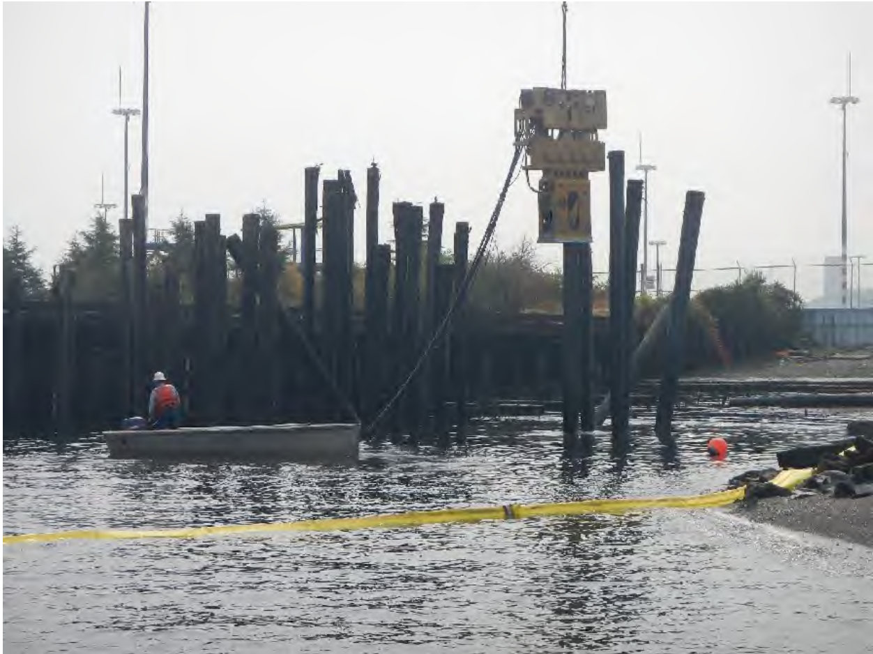
Photo 13 Vibratory Pile Extraction
