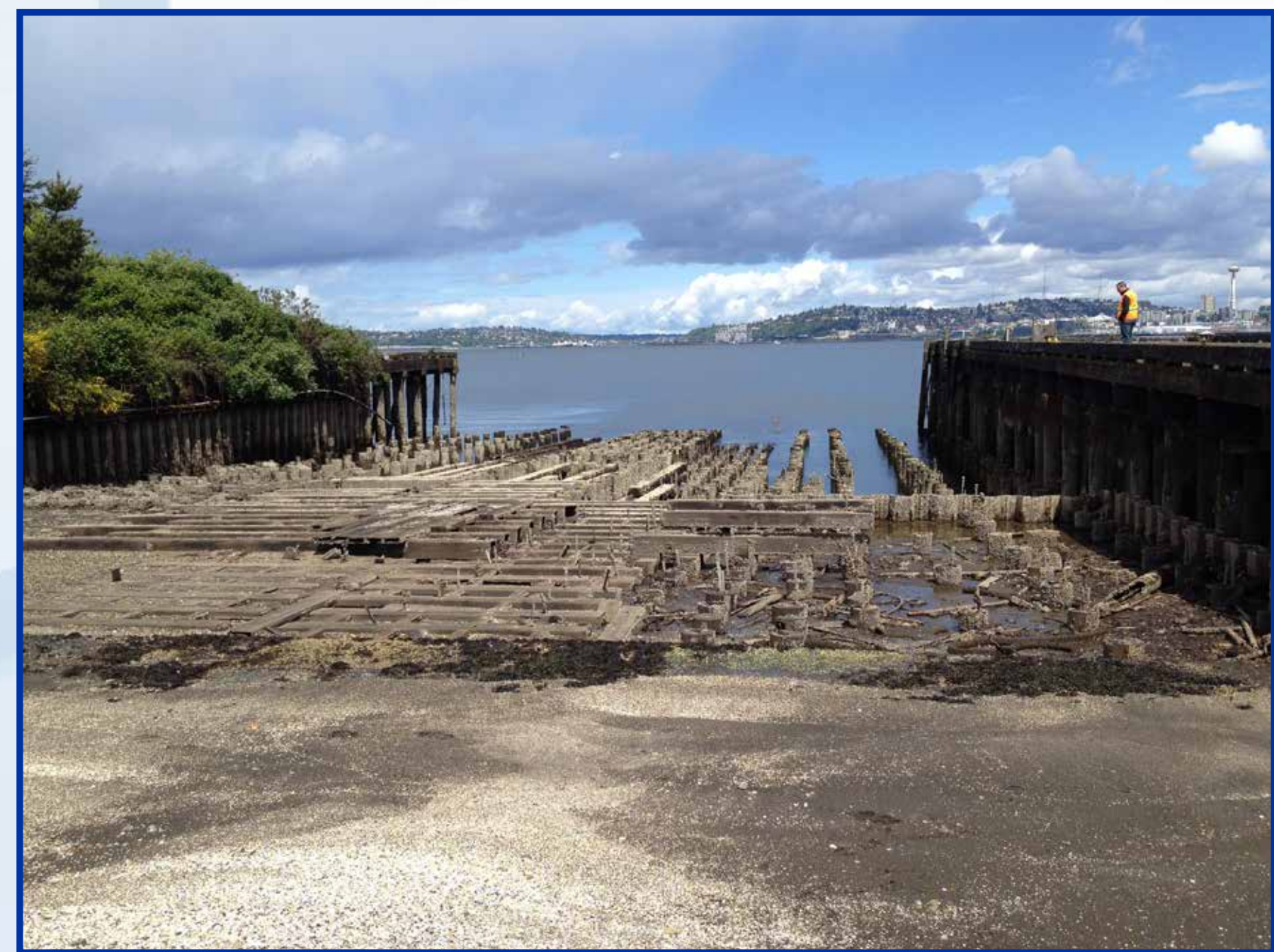
T 5 Shipway 2015 Before
