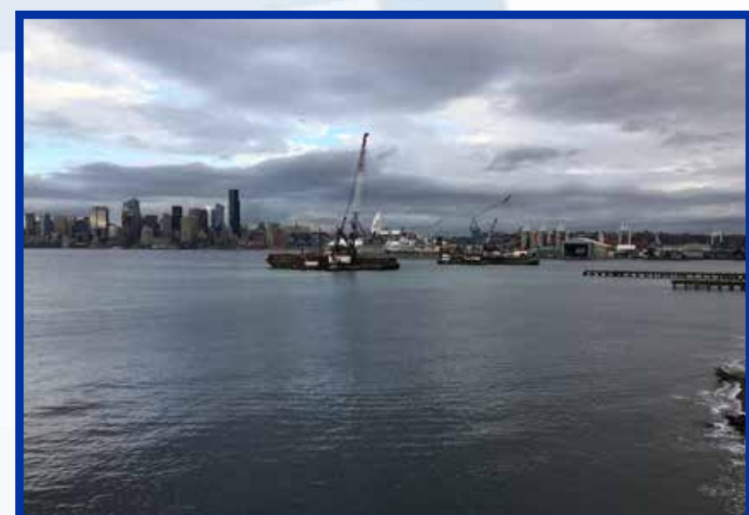
Dredge and fill platforms
