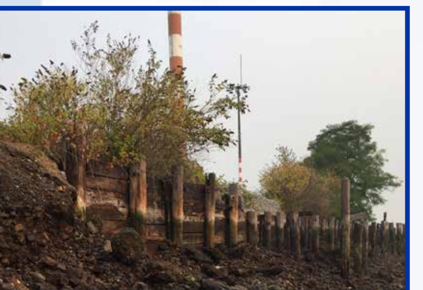
Lower tier bulkhead post removal
