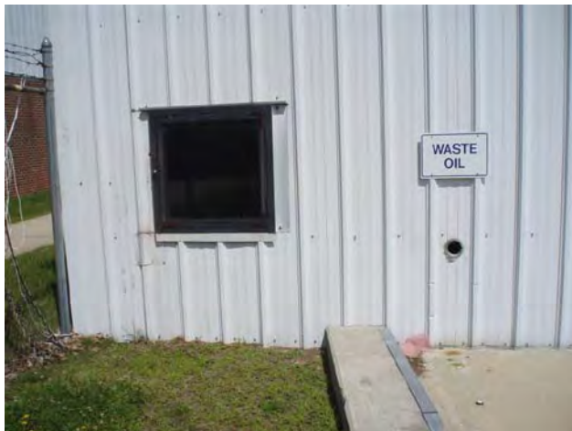
20.) Stoddard Waste Oil Delivery Area, Exterior
