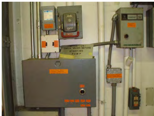
8.) Area 1 Trench At Hose Dispensing
