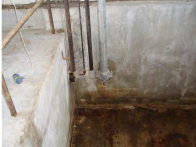
25.) Inside Oil House No Odor Tank Area; Inside Background
