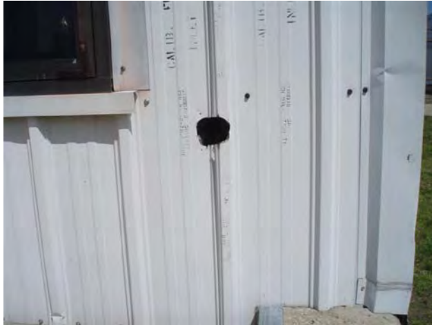
19.) Stoddard Waste Oil Delivery Area, Exterior
