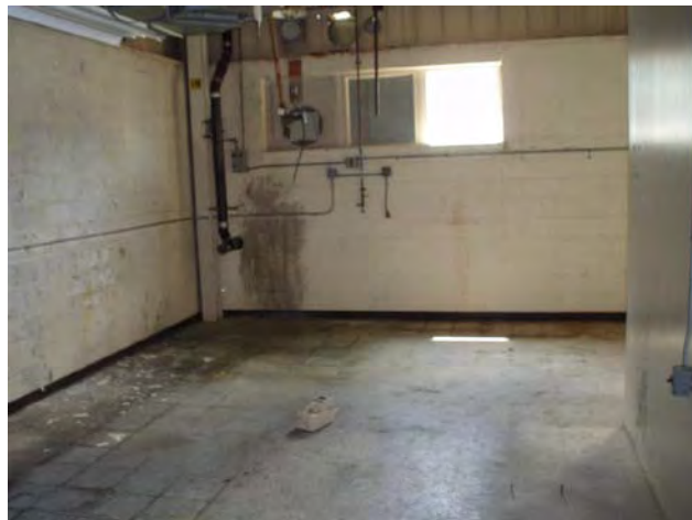
32.) Interior Rooms, Open Office C
