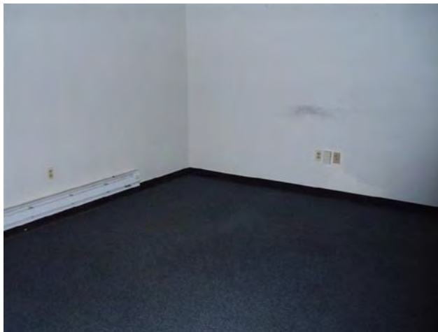
54.) Open Office B, Interior
