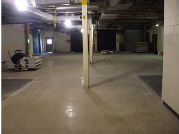
73.) Open Office D, Loading Docks
