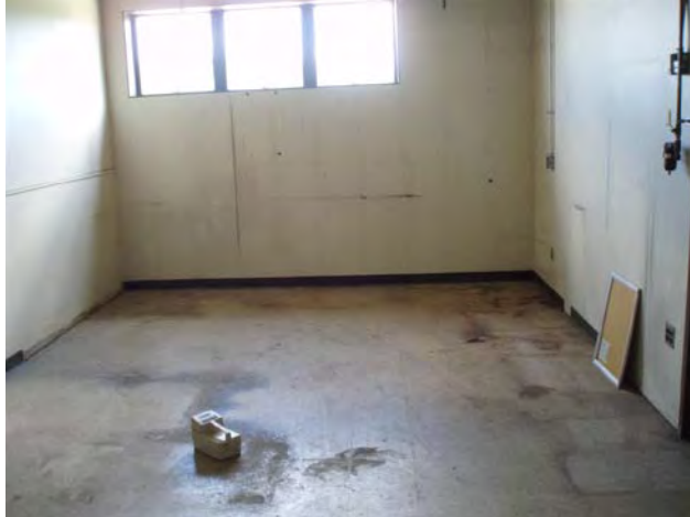
35.) Interior Rooms, Open Office C
