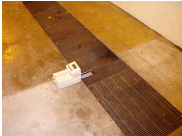
4.) Trench, Test Cell 3 (2.8 Ambient)
