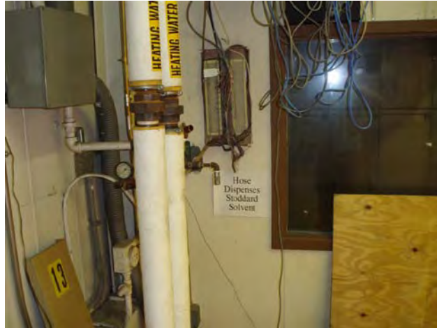
9.) Area 1 Trench At Hose Dispensing
