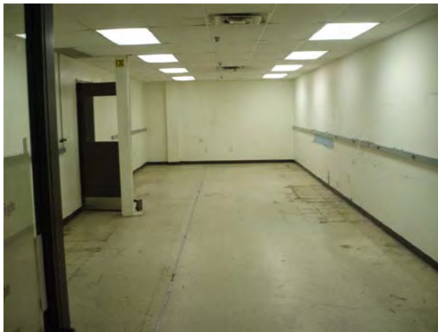
58.) Open Office B, Interior
