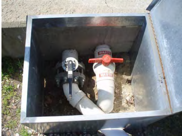
21.) Stoddard Waste Oil Delivery Area, Exterior
