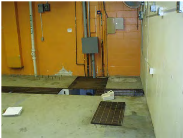
40.) Interior Rooms, Open Office C, Other Drain; Trench to BLDG. 3
