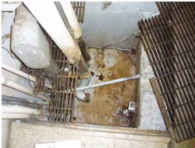
6.) Area 1 Trench At Hose Dispensing
