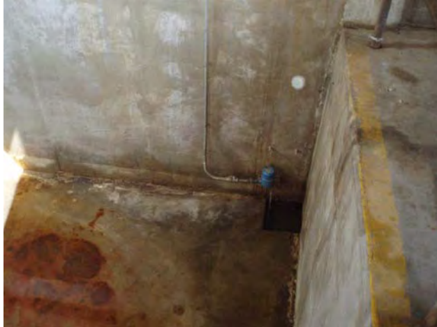
23.) Inside Oil House No Odor Tank Area; Inside Background
