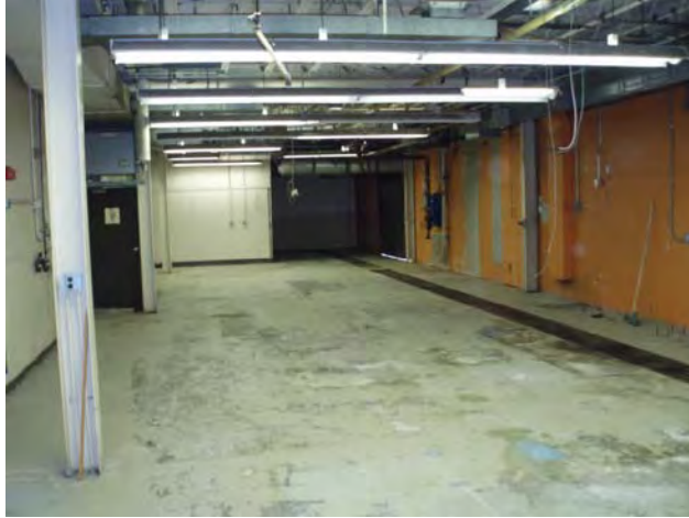
41.) Interior Rooms, Open Office C, Other Drain; Trench to BLDG. 3
