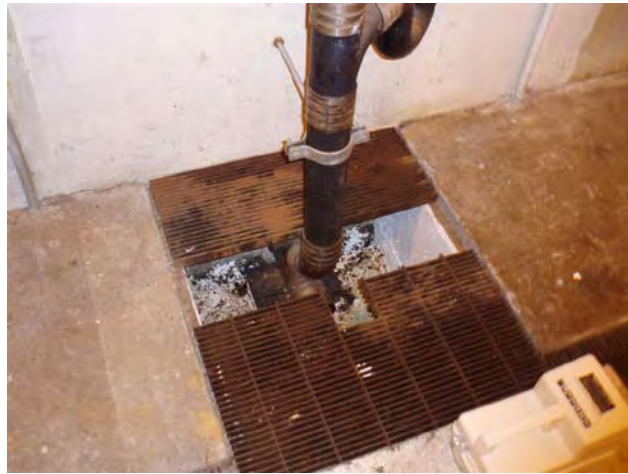
3.) Roof Drain, Test Cell 2 at Trench
