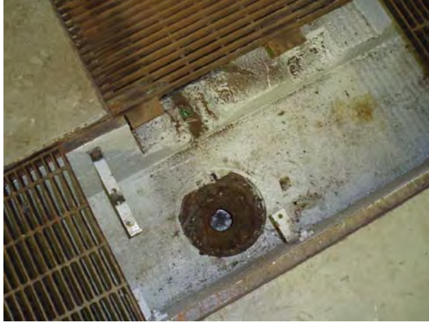
39.) Interior Rooms, Open Office C, Other Drain; Trench to BLDG. 3
