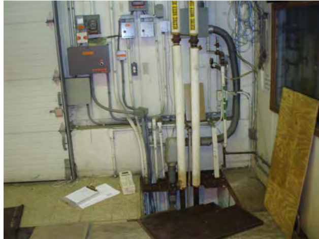
7.) Area 1 Trench At Hose Dispensing
