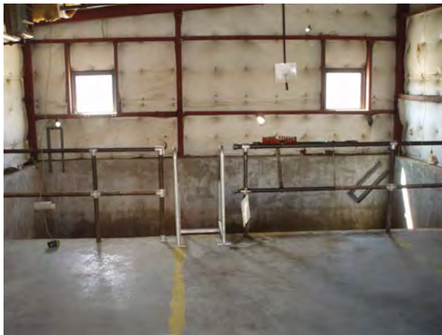
22.) Inside Oil House No Odor Tank Area; Inside Background
