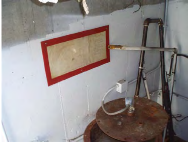
27.) Trench PUM Vent House Interior; Stoddard Odor
