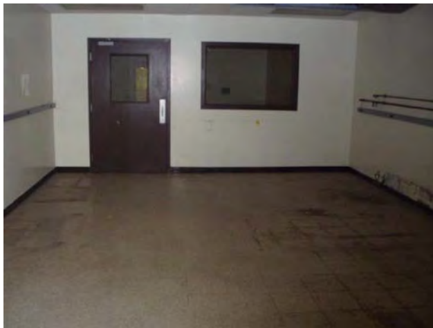
56.) Open Office B, Interior
