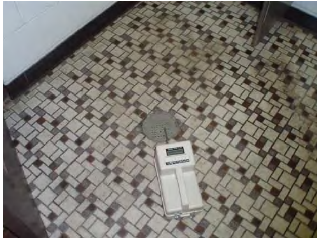
13.) Floor Drain, Bathroom
