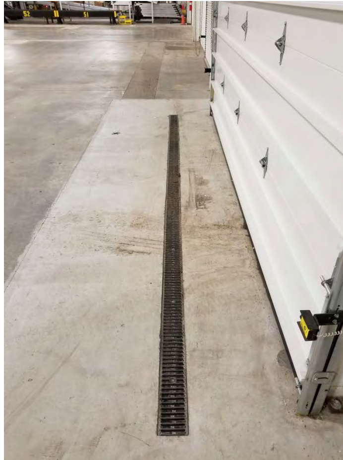
one of two trench drains at new overhead doors
