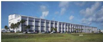
O&C BUILDING FRONT OR NORTHFACE VIEW
