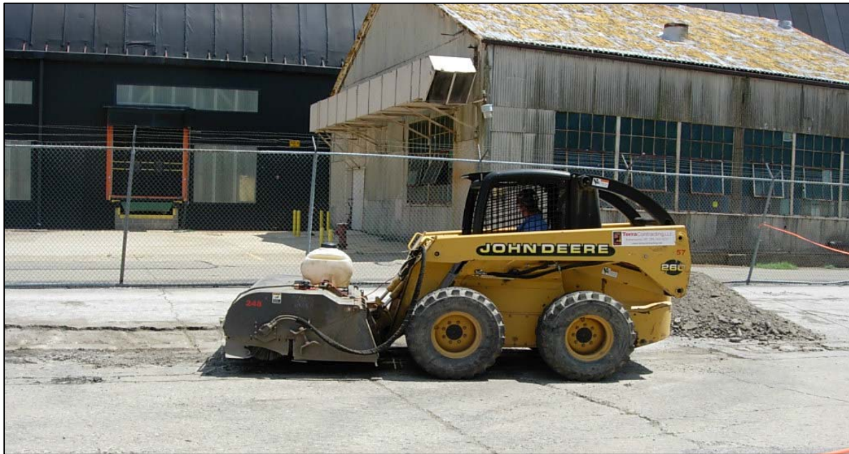
Photo 2 - Skid Steer debris removal operation
