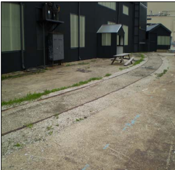
Photo 4a – Southwest Airdock door track before debris removal
